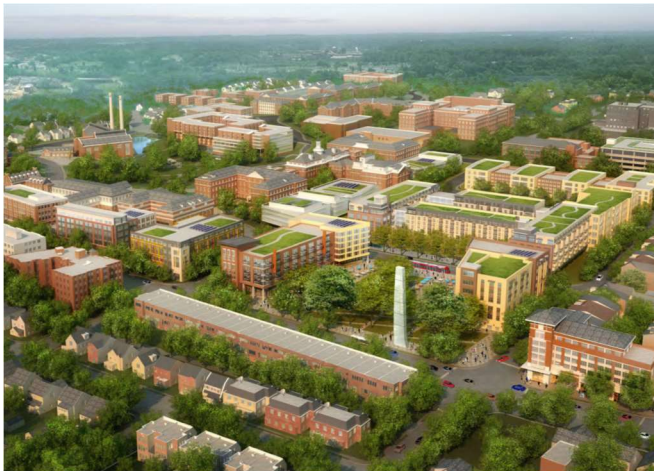
Walter Reed Redevelopment Project-- Original Hospital Building Upper Center
