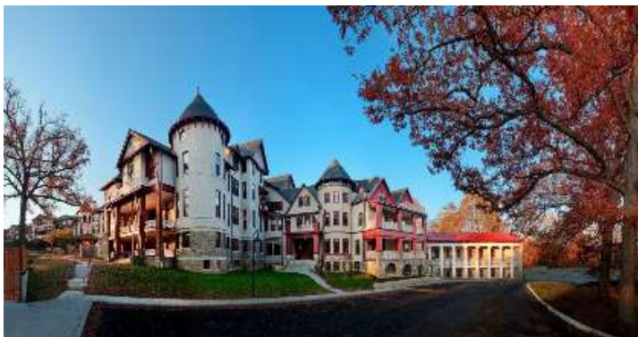
Forest Glen Main Building Renovation and Development
