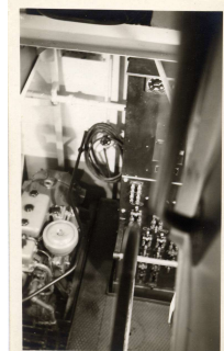
Engine room LCI 1033. One of eight GM diesel engines
